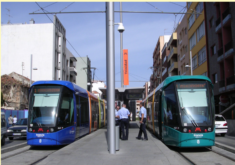
▼ The other end of the system is the La Laguna terminus, 7.5 miles from Santa Cruz. Here, two trams wait to return to the island capital. Both: Fred Landery
